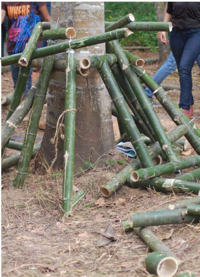
sample joineries “after completion
