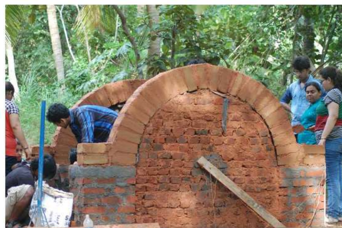
Completed arch opening using CSEB
